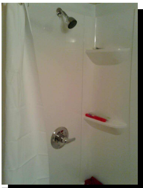
Workday installed a walk-in shower.
