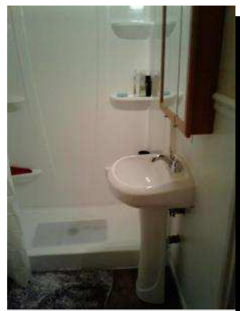
The bath redo included new fixtures.
